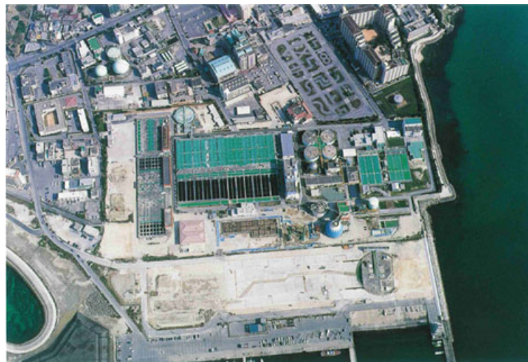
Fig. 2.1 Aerial view of NWTP.
