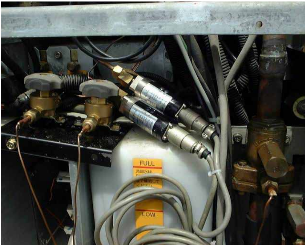
Figure A.13 Measurement of refrigerant pressure
