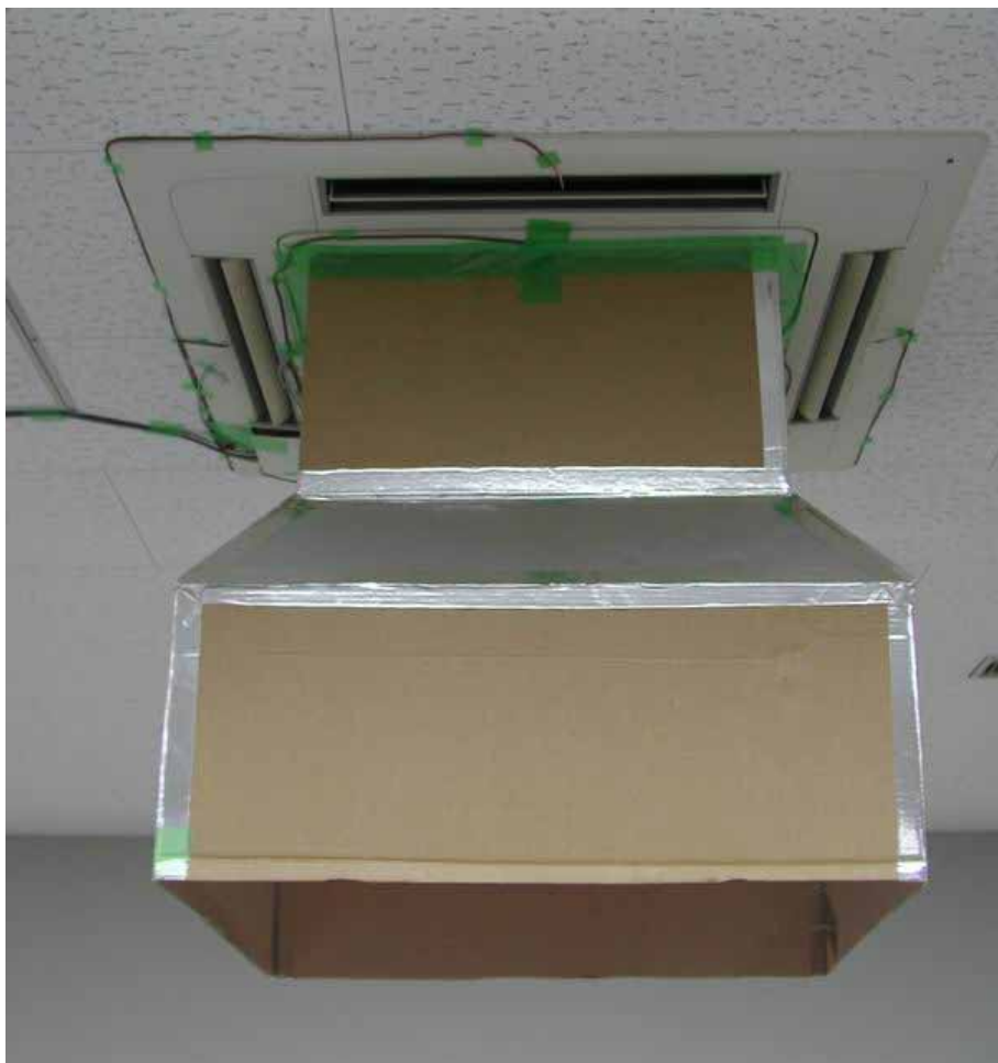
Figure A.9 Measurement of indoor unit air flow rate
