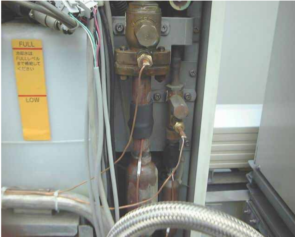
Figure A.12 Measurement of refrigerant temperature
