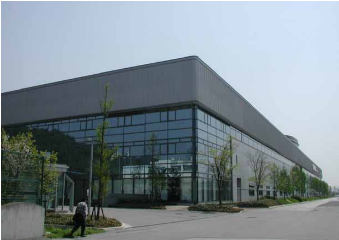
Figure A.1 Experimental building
