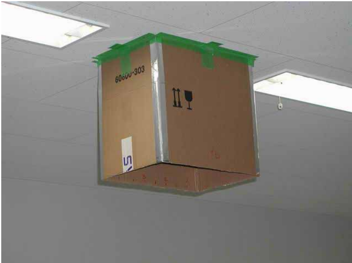
Figure A.14 Measurement of ventilation air flow rate
