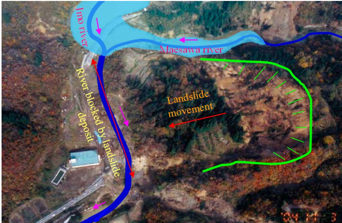
Plane view of the Higashi-Takezawa Landslide
