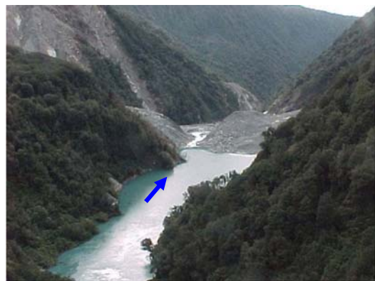
(f) October 24 th 1999: view downriver of the lake draining through the breached dam
