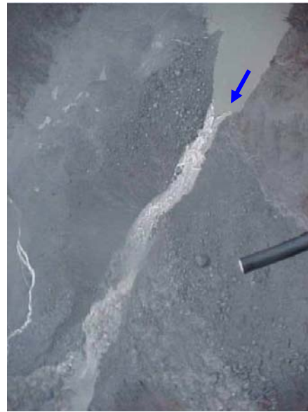
(d) October 12 th 1999: Vertical shot of the breach through the dam blocking the Poerua River after Mt Adams landslide
