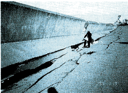
Photo 3 Top of the embankment of Yodo River
