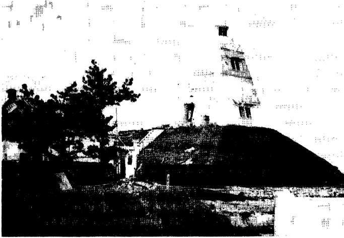
Photo 2 Lighthouse of Tenpozan in 1870s 35) .
