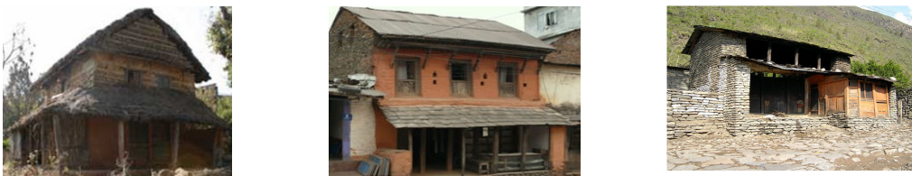
Fig.6.1 Typical stone masonry houses in Nepal
