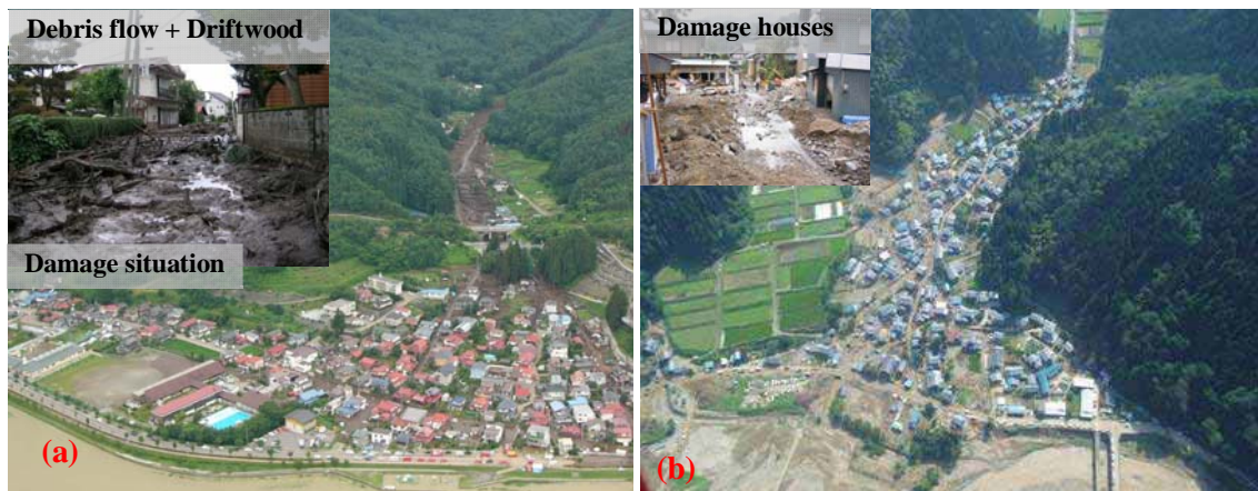
Figure 1.10 Debris flow disaster (a) at Odaizawa stream, Okaya, Nagano Prefecture, Japan, July 19, 2006, (b) at Miyama, Fukui Prefecture, Japan, July 18, 2004 (Photo Courtesy: Sabo department, MLIT, Japan)
