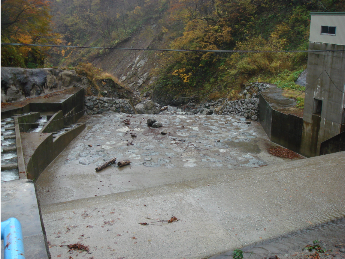
Figure 6.9: Weir at Okumotani station
