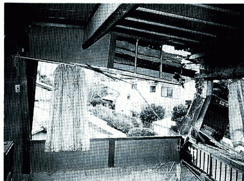
Photo 14 Pulling-out of column (second floor in the House TA).
