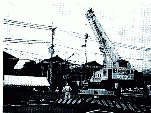
Photo 4 Loading test view using truck crane (House TU).
