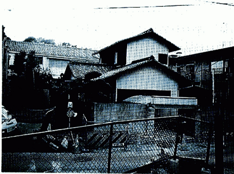
Photo 1 Earthquake damaged House SU (Nishinomiya).
