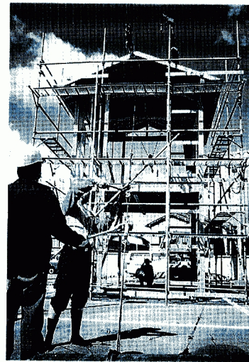
Photo 6 Free vibration test (Frame H).
