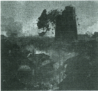
Photo 5 The brick construction structure which collapsed by the great Kanto Earthquake in 1923, described in the old postcard
