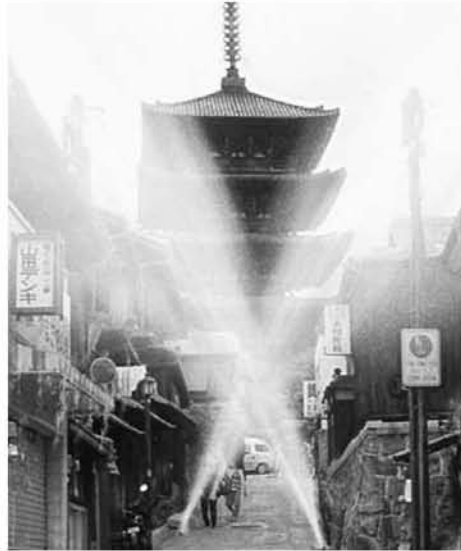
Fig. 13 Image of sprinkler system for narrow street (2nd fire-fighting phase) (Source: NPO for Protection of Cultural Heritage from Disaster, 2004)
