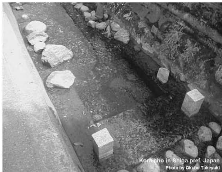
Fig. 5 A scooping pit for citizen's use (1 st fire-fighting phase)
