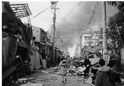
Fig. 2 A street of timber houses that collapsed in the Great Hanshin Earthquake (Source: AIJ)
