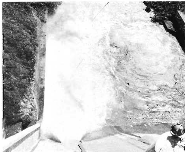
Fig. 14. Laterally back current at Tase Dam during one outlet operation.
