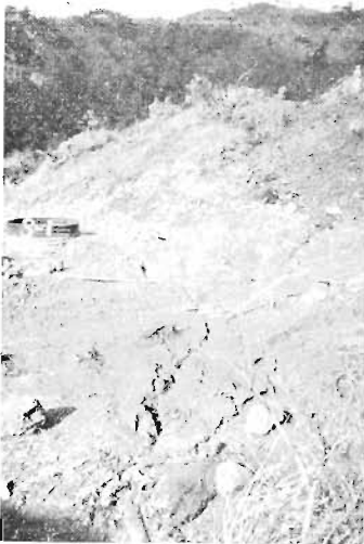
Photo. 7. Cracks occurred in the neighbourhood of Shaft No. 1.
