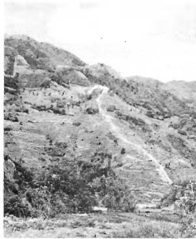
Photo. 1. Distant view of the neighbourhood of the penstock.
