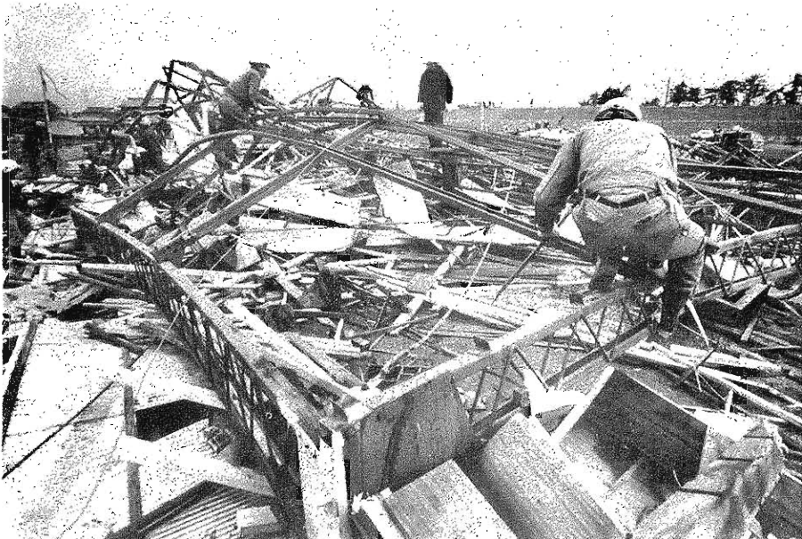
Photo. 3. Wreckage of a light-gauge-steel structure. Bodily removal of the structure from its foundations. (by courtesy of the Mainichi Newspapers)
