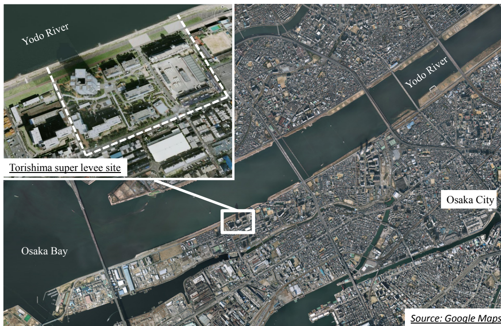
Figure 1.2. Aerial view of Torishima super levee site.
