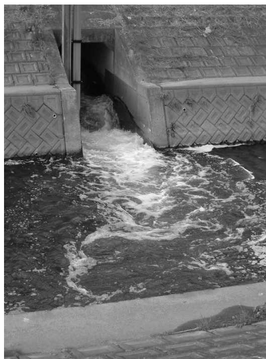
Photo 1 Uncontrolled release from a sewerage plant, causing an oily film on the surface, while kids were playing at the water.
