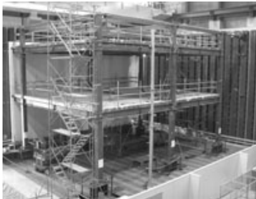
Figure 3: Overview of Test Structure (with ALC Panel)
