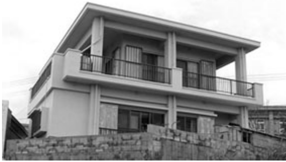
Photo 7. RC house with window shutters had few damage.
