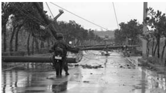
Photo 3. Broken electric and telephone poles prevents the traffic from passing.
