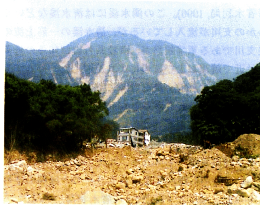
Photo 3 Debris flow disaster occurred at Junkeng district, Shangan village, Shuili, Nantou-ken (Many slope failures can be seen on the rear mountain)
