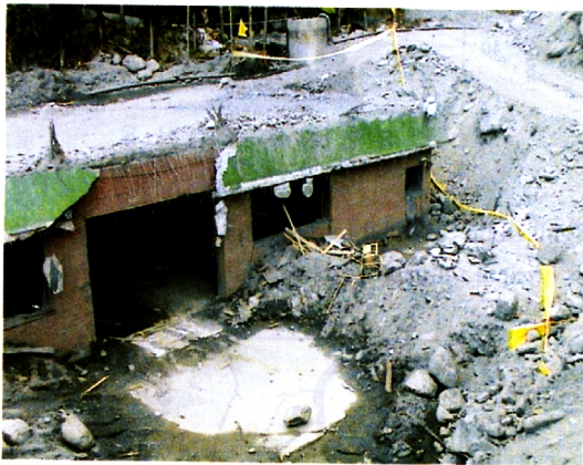
Photo 1 Baiyun mountain cottage buried with sediment by a debris flow occurred at Daxing village in Hualien-ken
