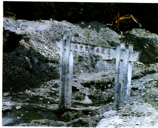
Photo 2 Stone gate buried with sediment by a debris flow at the entrance of Shuiyuandi district, Fengyili village, Fenglin, Hualien-ken
