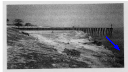
Pile dike along the Jamuna (Klaassen, 2002).
