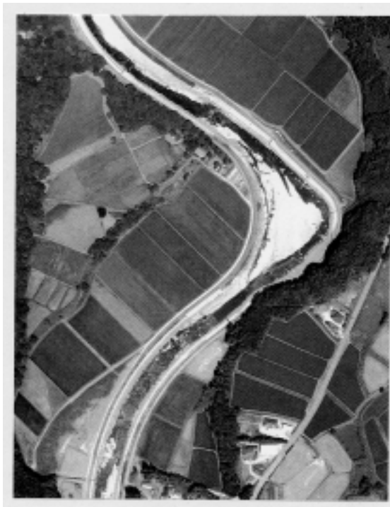
Photo 7 Aerial photographs taken after the river improvement work around the curved channel in upstream area of Hosihata district
