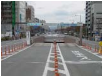
Photo 1 Entrance of underground parking lot
