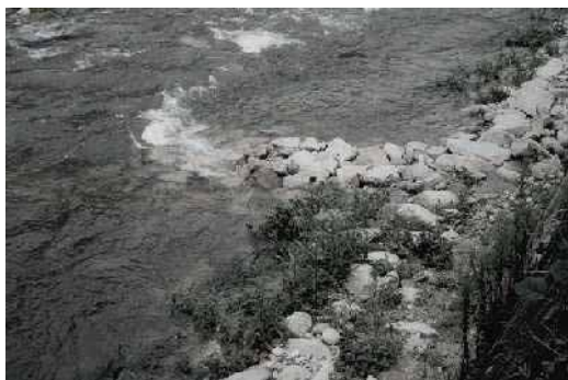
Photo 3 Rubble mound groin in Akechi River
