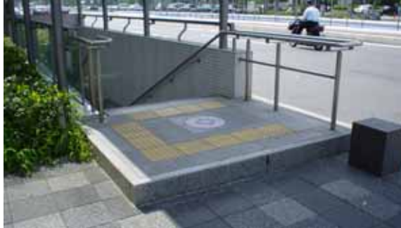
Photo 3 Entrances to Oike underground space. (top :Car entrance, bottom :Pedestrian entrance )
