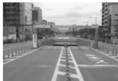
Fig.16 Entrance of underground parking lot
