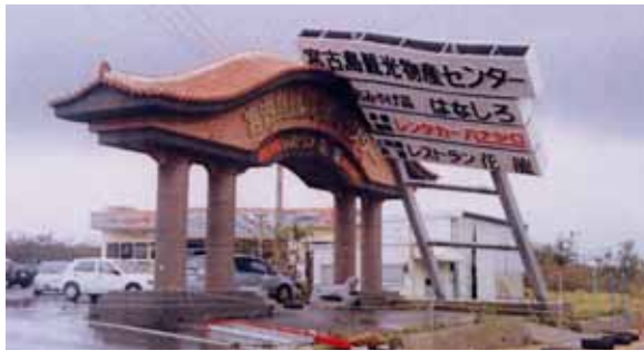
Photo 9 Inclined AD tower (courtesy Okinawa prefecture branch office)
