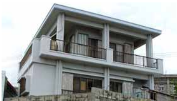
Photo 32 RC house with shutter on the windows
