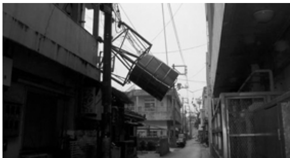
Photo 11 Fall of water tank (courtesy Hirara Tsutomu)
