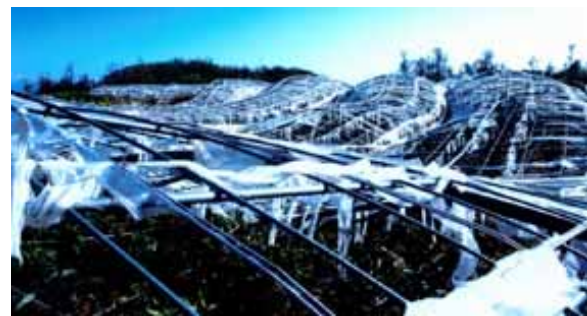
Photo 14 Damage of vinyl houses (courtesy Nougyousevenjo Miyakosijo)
