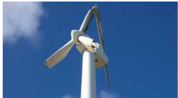
Photo 20 Broken blades of wind turbine ( Okuda et.al. 2003 )
