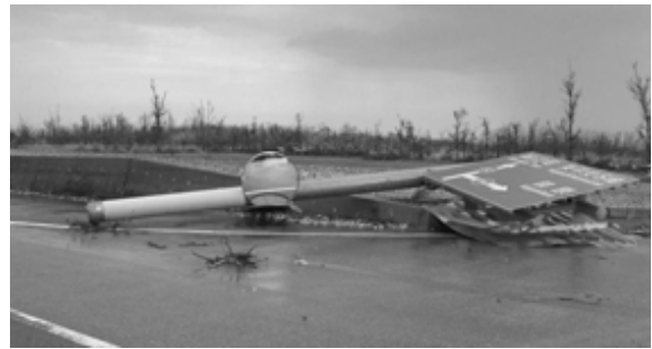
Photo 10 Break of road signs (courtesy Hirara city)
