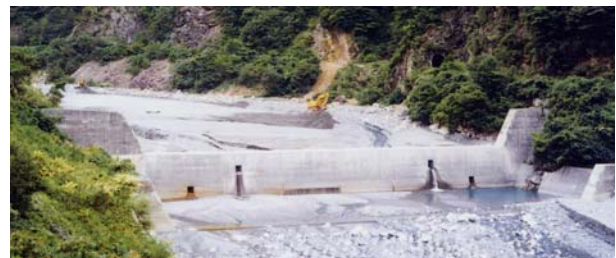
Photo 1 Upstream check dam of Koshibu dam Japan (Sumi et al., 2006)
