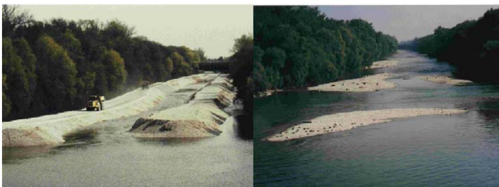
Photo 10 Gravel replenishment into Isar at the Oberföhringer Wehr: Transport of excavated material by truck and deposition in the river bed as depots (left) and naturally distributed gravel material after minor flood events after 3 months (right) (ALPRESERV project)
