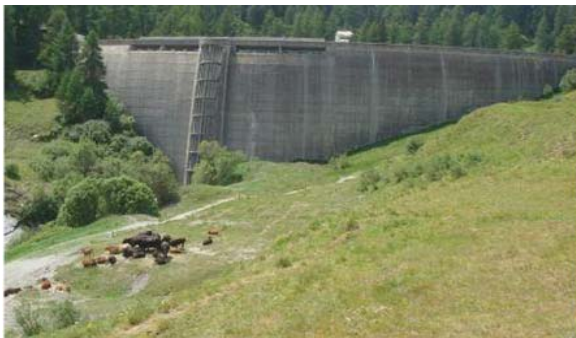
Photo 7 Flood retention basin of Orden dam, Switzerland
