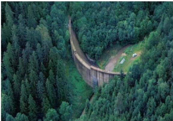
Photo 6 Flood mitigation dam of Ligistbach, Styria, Austria
