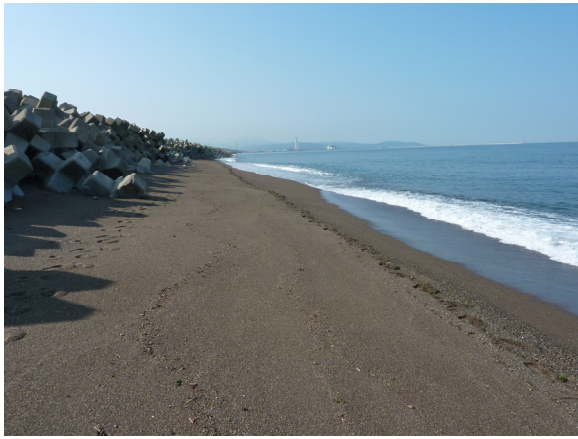
Photo 1 Shore line in front of wave dissipating concrete blocks at the location of the old observation pier
