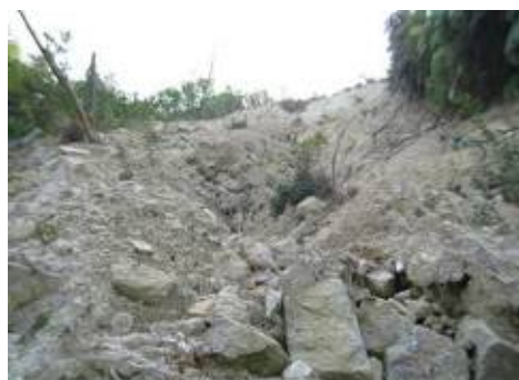
Photo 2 Collapsed slope in Manao, Hohfu city, Yamaguchi prefecture
