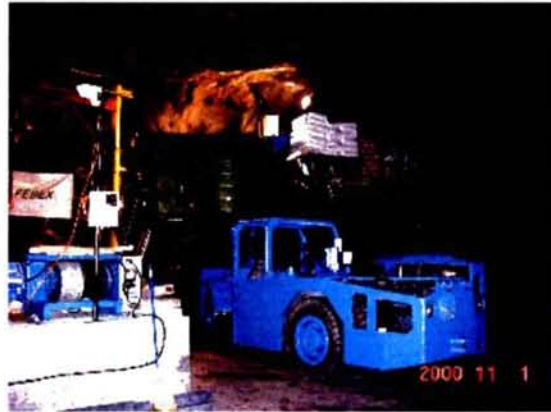
Figure 5.15 充てん材の練り混ぜ状況
