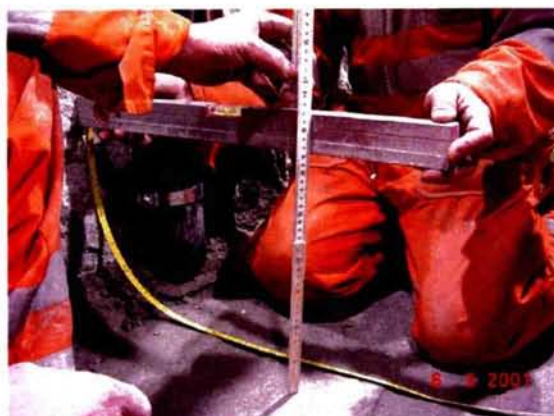
Figure 5.18 締め固め後の高さ確認
