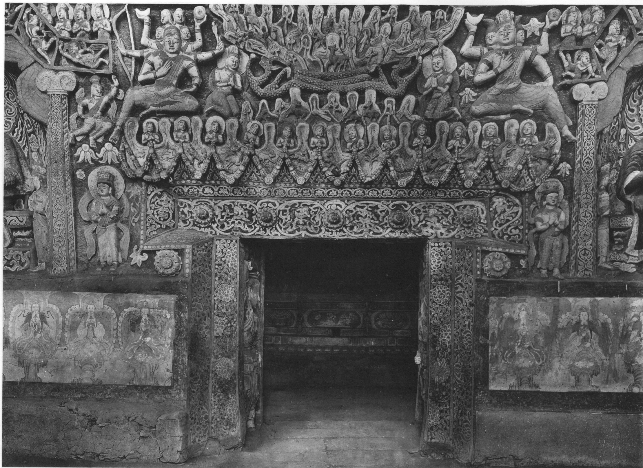
Ante-Room, North Wall, Entrance Gateway.
