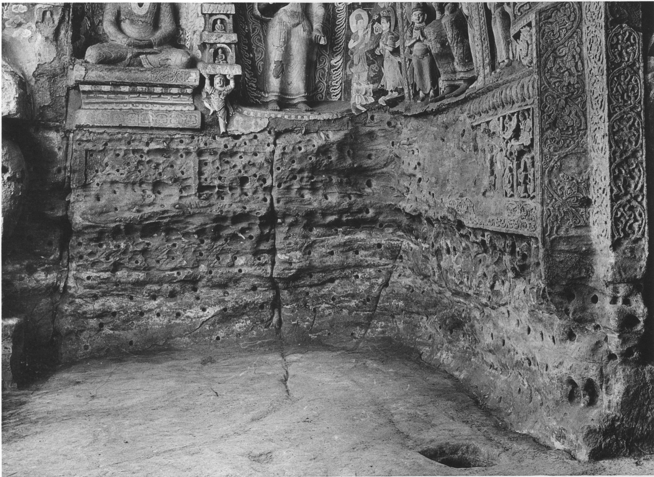
Ante-Room, West Wall, Bottom Storey.
