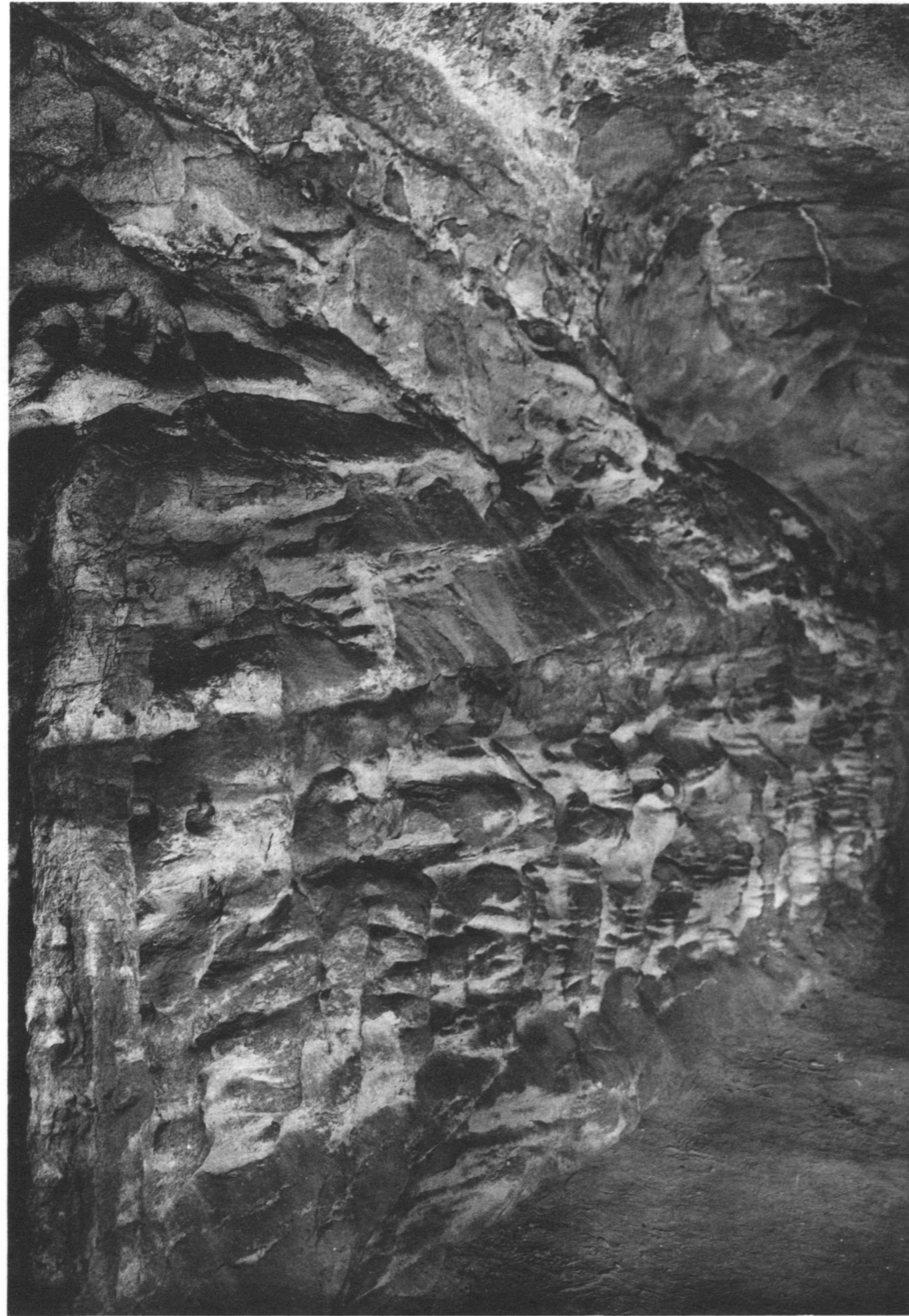
A) Passage, South Wall. 隧道 南壁
