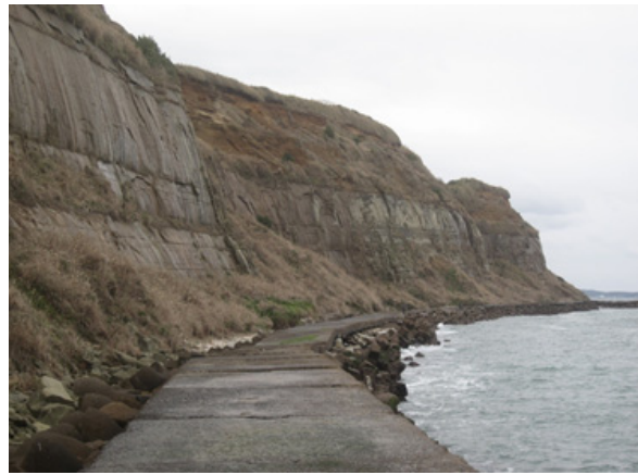
Photo. 1 Sea cliff with shore-protecting dyke, Byobu-ga-ura, Chiba (photograph 16 December 2009)
