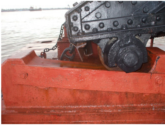
Photo 3 Connection of floating small pontoon and Bridge
