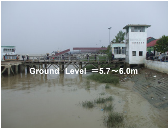
Photo 1 Relation of pier, seawall and road
