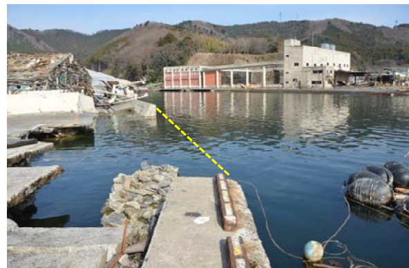
Figure 10 Lost sea walls in Onagawa fishery port.
