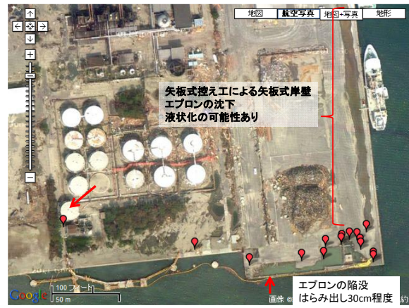
Figure 4 Satellite image of damaged area in Nakajima wharf.
