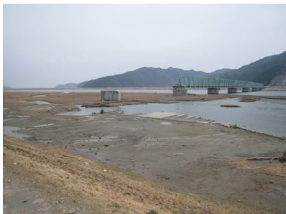
Figure 12 View of the Shin Kitakami bridge.
