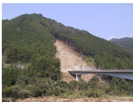
Photo 1 upper) debris flow hit a house in Minamata, Kumamoto Pref.; and lower) shallow landslide in Miyagawa, Mie Pref.
