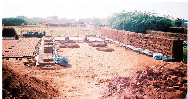
Fertile soil/being used for brick making work
