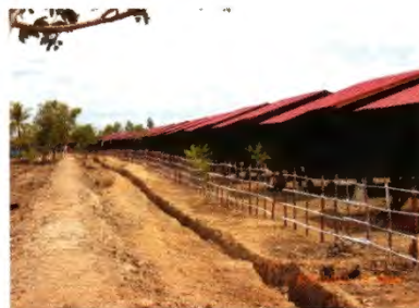
Construction of rural houses
