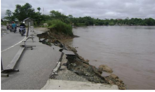
Photo 2 Mass failure on Sesayap riverbank
