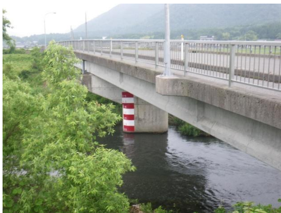
Photo 5 The simple graduated staff gauge at the Ane River
