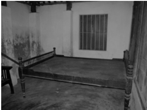
Figure 15. Chai Dong is not used and has fallen into disrepair
