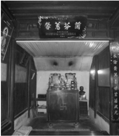
Figure 14. PVC ceiling used to protect worship space in Nha Chinh
