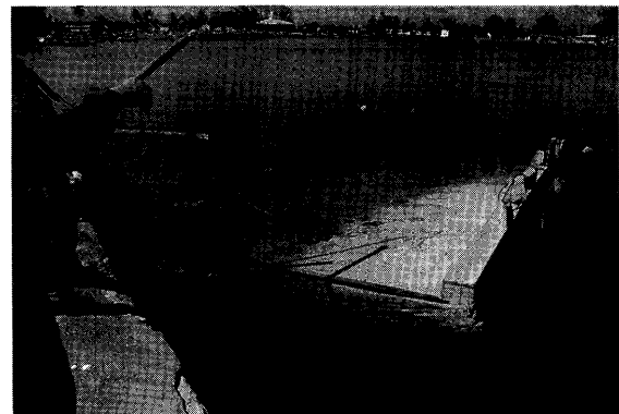
Fig. 15 Collapsed floor slab of a passenger jetty at a ferry port in Ujung Kalang, Meulaboh)
