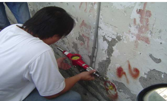
Fig. 7 Measurement using tape extensometer
