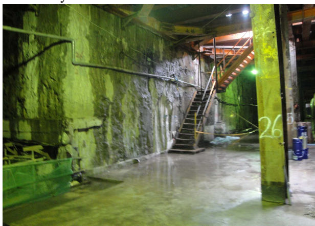
Fig. 3 Quality of diaphragm wall
