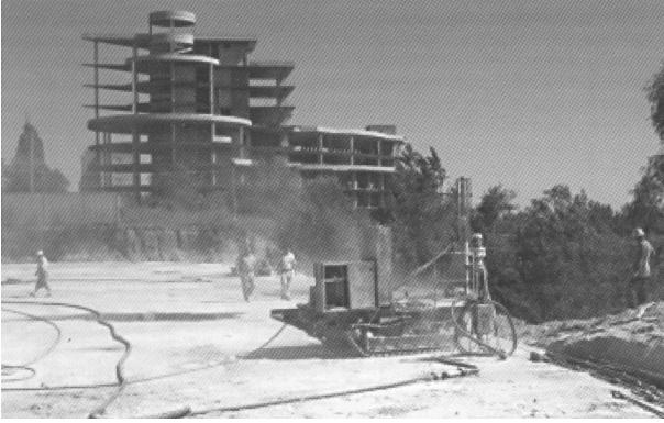
Figure 4. Drilling of cement chinks
