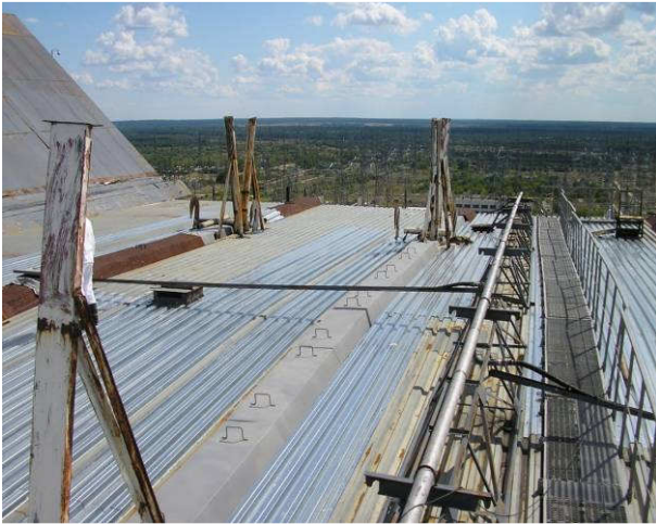
Fig. 10. Repair of the light roof (measure w/n)
