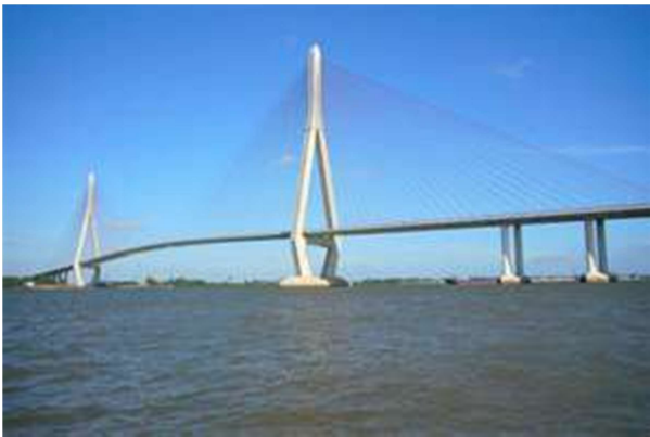
Fig.19 Can Tho Bridge after completion
