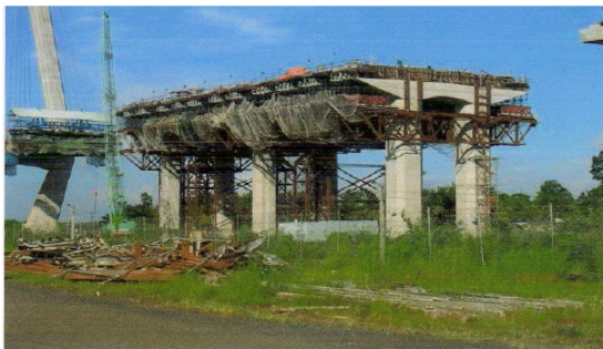
Fig.13 Construction view before collapse
