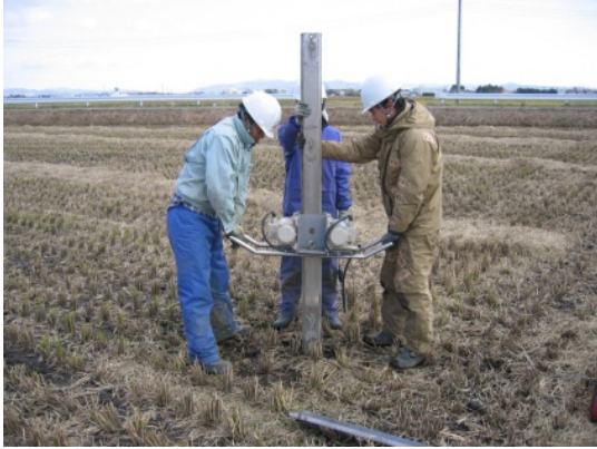
Fig. 2 Working scene of coring survey by using Geo-Slicer.
