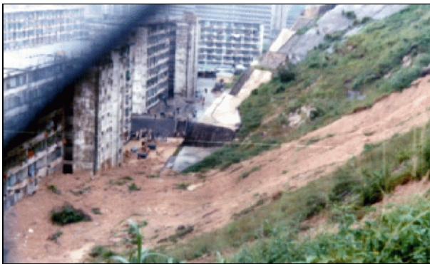
Figure 1 Sau Mau Ping slope failure: view behind Block 9 (Binnie and Partners, 1976)
