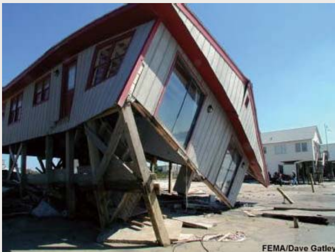
(b) Destruction from storm surge (Source NOAA)
